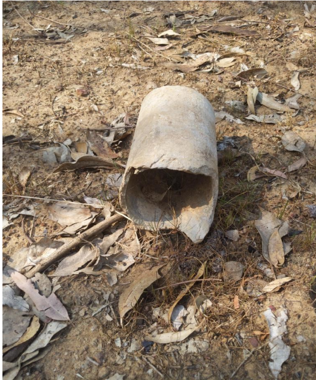
Photo 5 - Potential ACM Pipe
